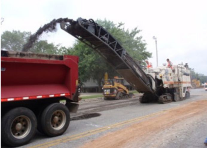
Removal of a controlled thickness of asphalt pavement using a milling machine.
