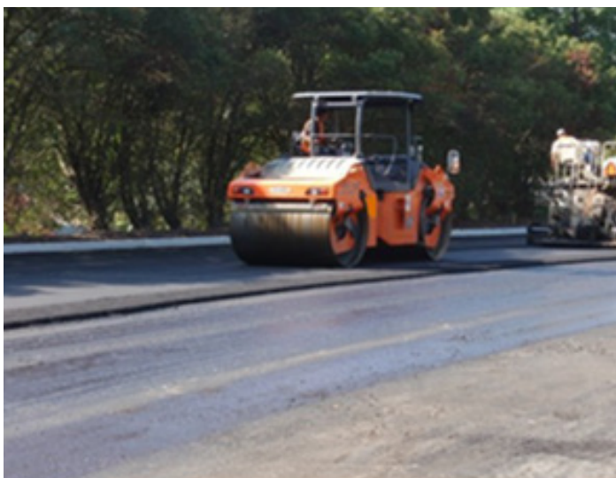
Initial breakdown compaction of an asphalt surface course.
