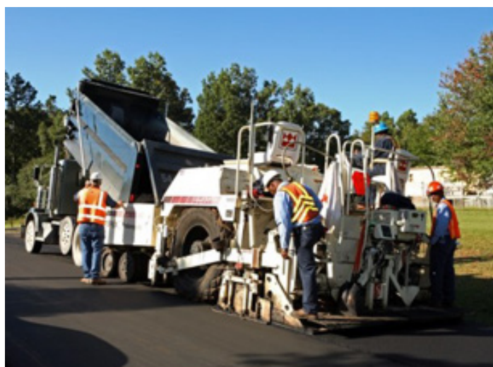
Placement of an asphalt overlay.
