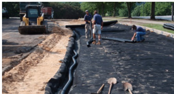
Installation of a pavement underdrain.
