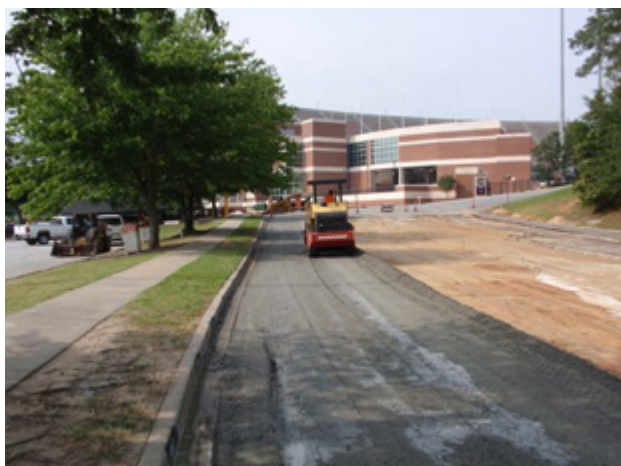
Preparation of subgrade and aggregate base course.
