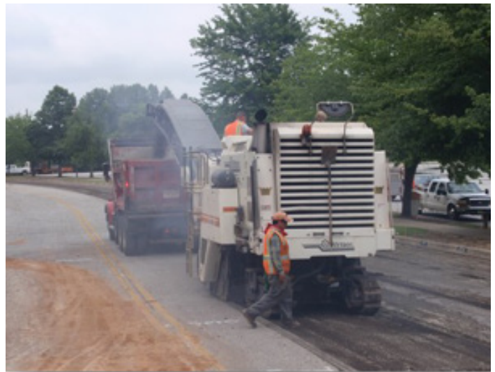
Milling an existing asphalt pavement.
