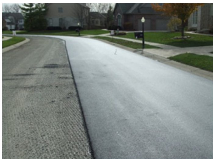
Newly placed asphalt overlay.
