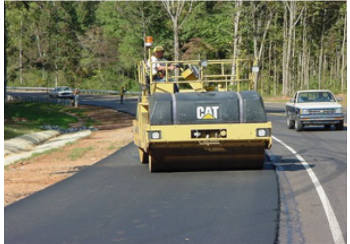
Compaction of an asphalt overlay.
