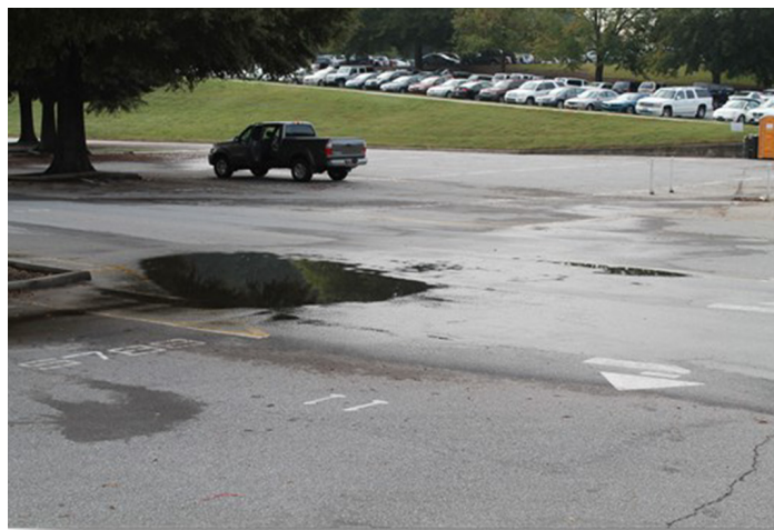
"Bird bath" due to inadequate pavement slope
