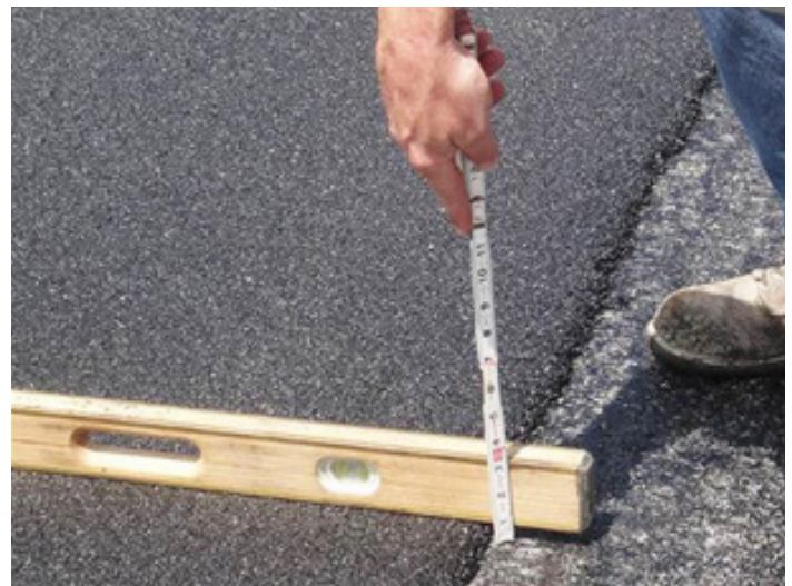
Thin lift asphalt overlay(Thinlay).
