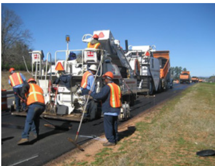
Placement of an asphalt surface course.
