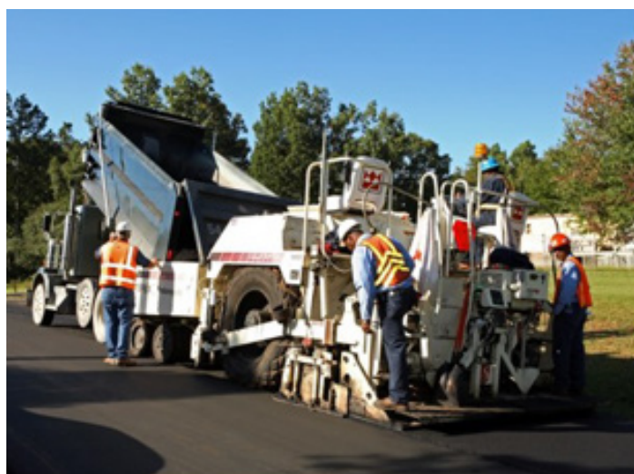
Placement of an asphalt overlay.
