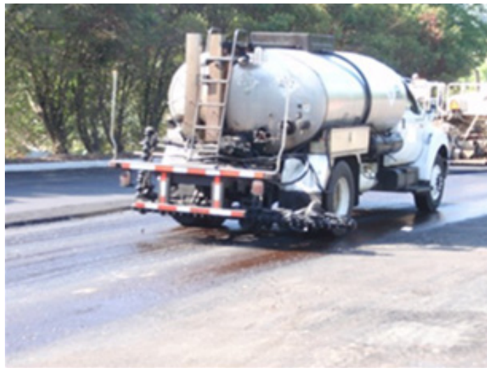
Application of a tack coat prior to paving.
