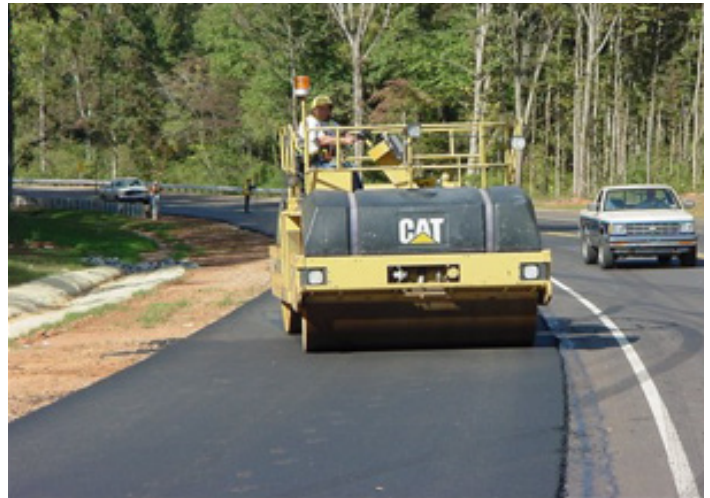
Compaction of an asphalt overlay.
