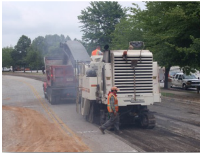
Milling an existing asphalt pavement.
