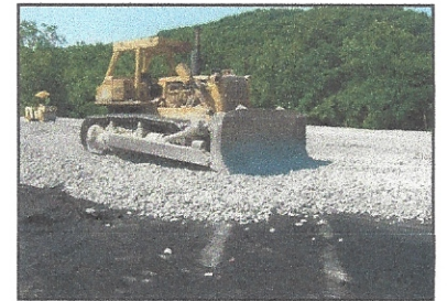
Figure 4 - Dozer spreading aggregate reservoir layer on Non-Woven Geotextile Filter Fabric.
