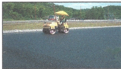
Figure 9 - A small roller compacting the pavement.
