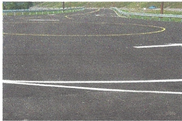
Figure 10 - The standard dense graded asphalt entering the parking lot.
