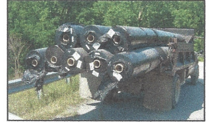
Figure 2 - Truck delivering the Non-Woven Geotextile Filter Fabric.
