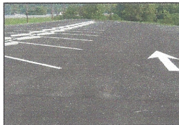
Figure 11 - The porous asphalt section of the parking lot
