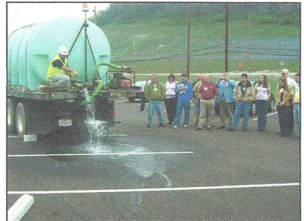
Figure 12 - A demonstration shortly after the porous parking lot was installed.
