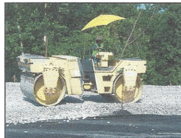
Figure 5 - Roller leveling the surface.
